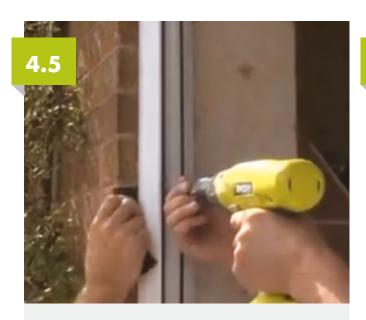
Fix the side of the frame to the wall. Use packers at the fixing points to avoid distortion to the frame and to maintain the 5mm expansion gap.
