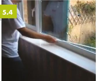
Make sure the area is clean and free from dust and debris. Measure and fit any internal trims that may be required. Trims maybe fitted using a suitable PVC-U adhesive or silicone.
