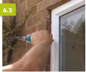
Apply a strip of masking tape to the frame perimeter. Apply a smooth bead of silicone sealant between the frame and brick work. Before the sealant sets, remove the making tape to create a neat finish.
