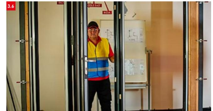
➤ 3.6 Test the operation of the door to ensure it runs smoothly.
