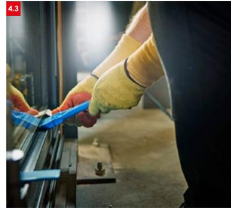
➤ 4.3 Position 2 packers, one inline at the corner that is to be toe and heeled with the other at 90° on the opposite side.
