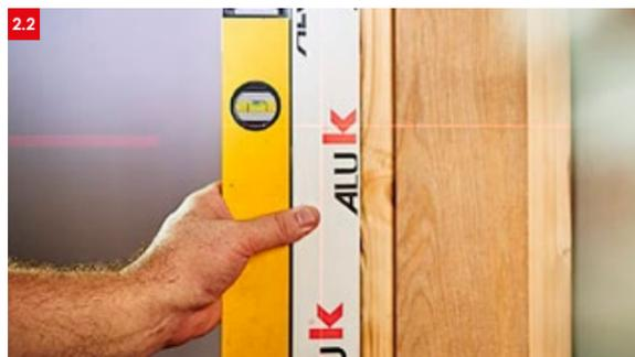
➤ 2.2 Ensure the frame is plumb. Again, a laser level is useful to achieve this.
