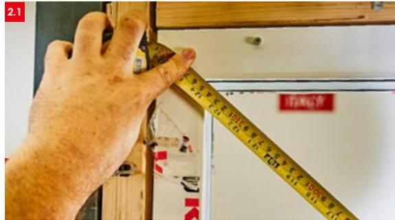
➤ 2.1 Offer the frame into the opening and check for squareness by measuring the diagonals. There should be no more than 2mm difference between them.
