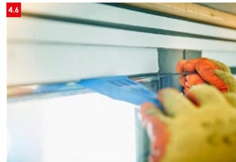
➤ 4.6 And the top corner which is diagonally opposite to the glass packing at the bottom.
