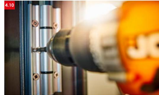
➤ 4.10 **Important!** Once the door is operating correctly and the 12mm gap top and bottom has been maintained, lock off by fitting 4.2 x 25mm stainless steel countersunk self tapping screw to rollers, guides and hinge. If the frame and doors arrive as an assembled unit check to see if these locking screws have been fitted in the factory.
