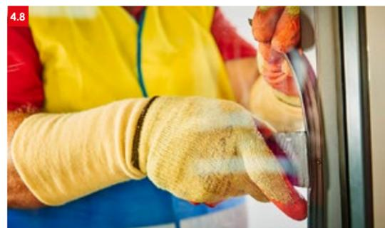
➤ 4.8 With weak soapy water (if required) fit the wedge gasket in one piece. Remember to force into the corners first and then loop from the centre towards the corners (if necessary snip the bottom of the gasket to facilitate ease of fitting at the corners) Ensure the wedge gasket is not stretched and is cut oversize by 10mm per meter.
