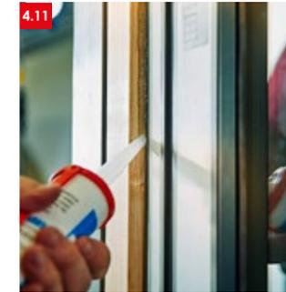
➤ 4.11 Seal perimeter with proprietary sealant. Be sure to follow sealant manufacturers instructions regarding backer rod and primer.
