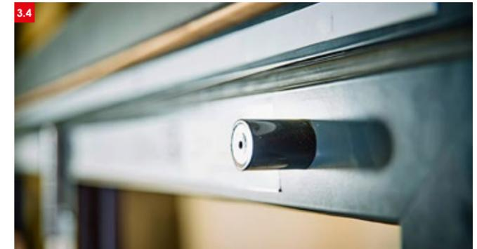
➤ 3.4 Check that the traffic door magnets have been fitted and that they align when in the open position.
