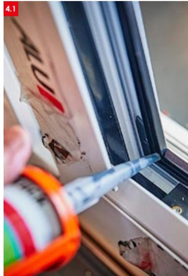
➤ 4.1 Check the captive glazing gasket to ensure it has been fully fitted with no gaps at the corners then seal the corners with a butyl based sealant.
