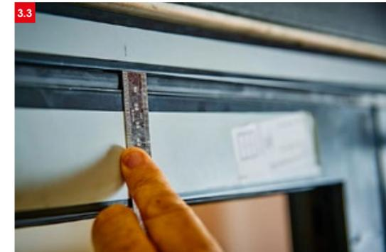
➤ 3.3 Ensure that there is a 12mm gap top and bottom between the outer frame and the door panel.
