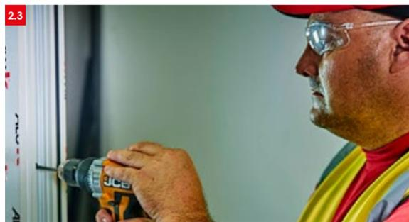
➤ 2.3 Don't forget, fixing centres should be 100 - 150mm in from each end and a maximum of 600mm thereafter.
