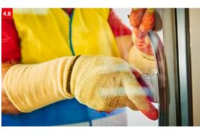
corners first and then loop from the centre towards the corners (if necessary snip the bottom of the gasket to facilitate ease of fitting at the corners) Ensure the wedge gasket is not stretched and
