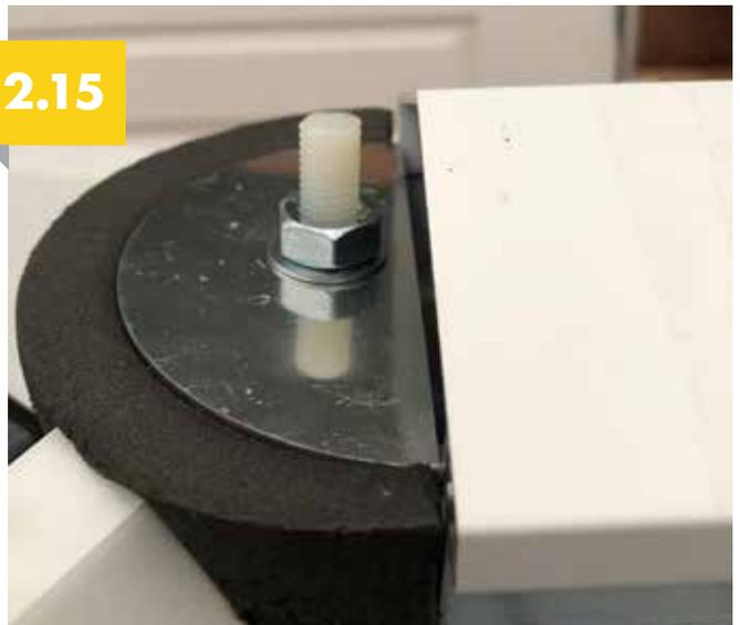
Fit the foam bung and clamp plate and tighten M10 nut until the foam is firmly pressed down onto glazing.
