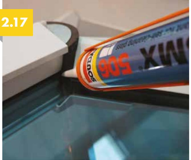
Seal around perimeter of the foam bung where it intersects the ridge glazing seal, glass and glazing bar top caps.
