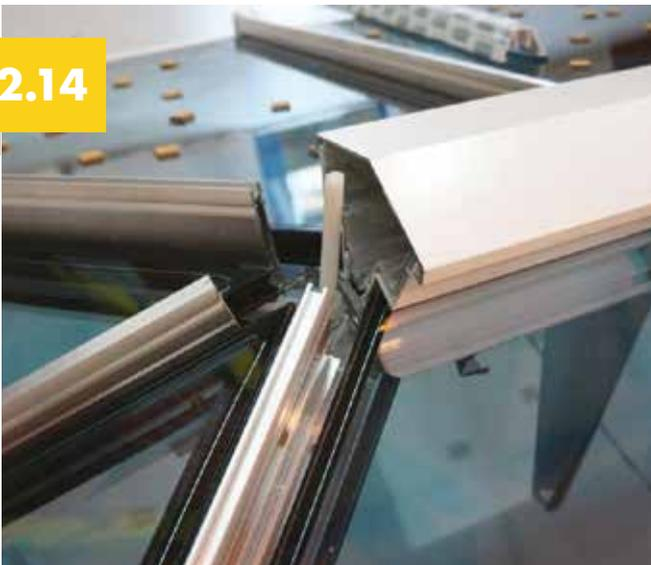
If not already fitted, fit the glazing bar end caps and glazing stops. Then peel back two inches of eaves beam seal tape film and fold to the outside. Insert glazing unit ensuring equal coverage and ensuring the glass is resting onto the glazing stops.
