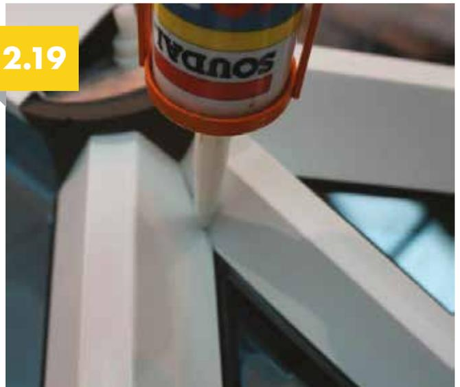
Seal the rafter top cap to hip top cap from the gasket intersection to foam bung.
