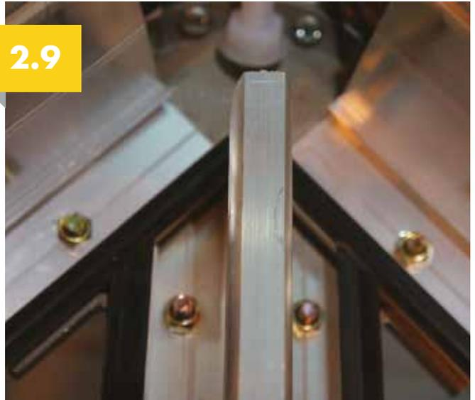
Fasten the central rafters to the spider using 1 x CRS8625S double stud and nuts. If jack rafters are present, please refer to Section 3: Installing Jack Rafters on page 10.
