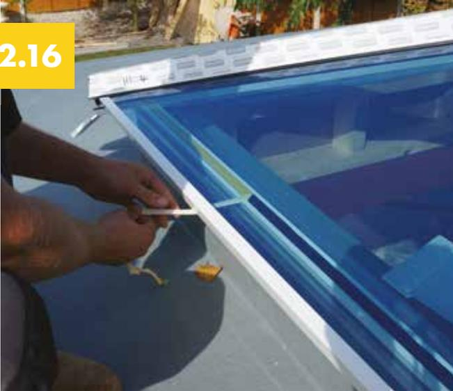
Fit the rafter and hip top caps using a nylon mallet, then ensuring the glass is positioned correctly, peel the remaining eaves beam seal tape film away and press glazing down to ensure contact with eaves tape.
