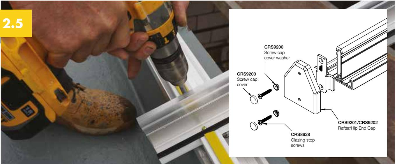
If access to the bar ends is limited, it is advisable to fit the glazing stops and end caps as shown (right) before fixing rafters to the ring beam. You can then proceed to loosely secure the side rafters to the ring beam using the threaded studs located down the ring beam.
